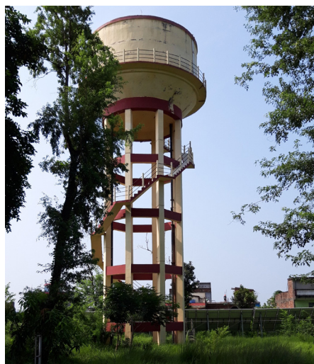
Elevated water tank.
